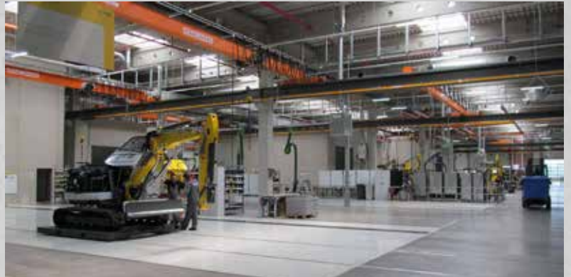
Industrial hall 50000 m 2 reinforced only with Fibrofor High Grade, jointless
