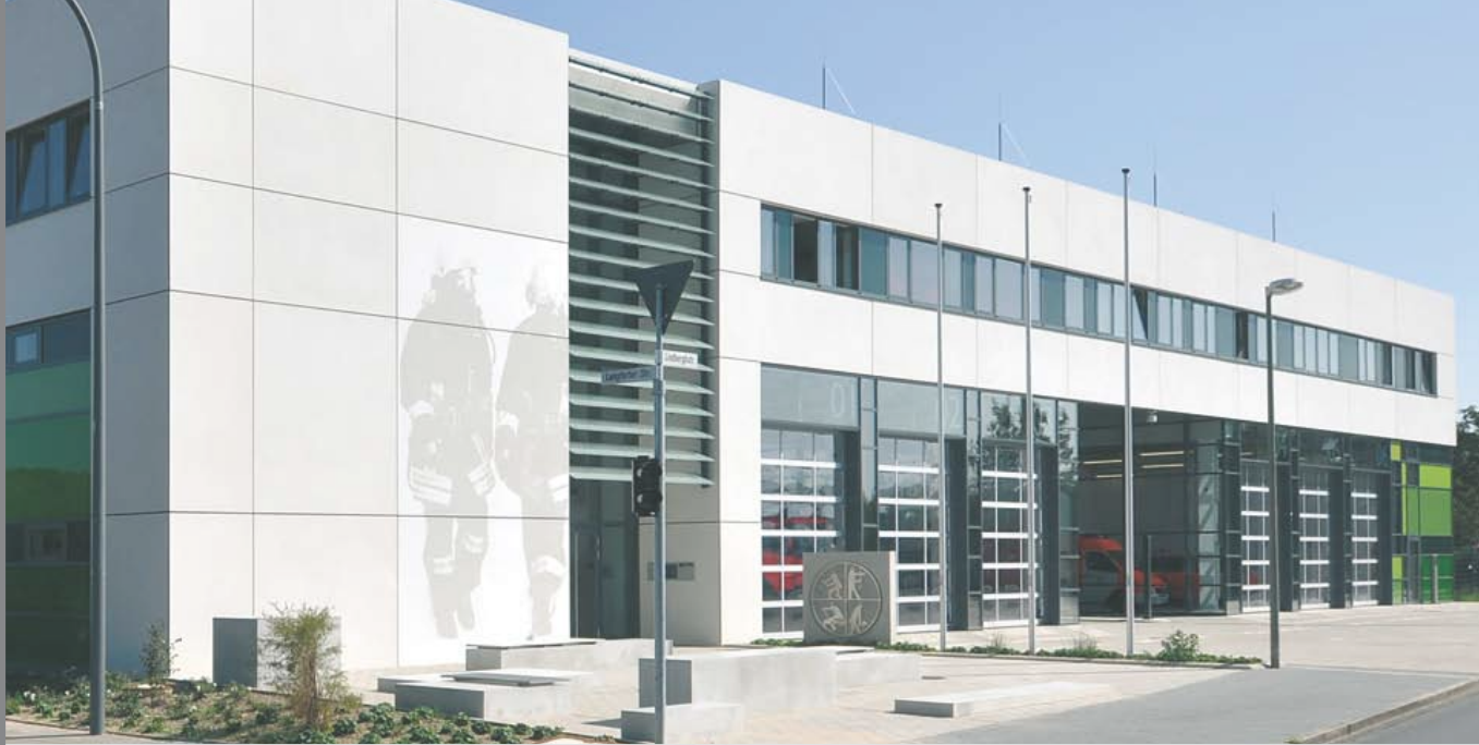
Photo: BetonBild, Facade: Hering Bau
